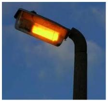
produced. Switch on times were therefore set to allow the lamp warm up to be completed when the light was needed. LED lamp switch on is instantaneous and by removing the warm up period we can switch lights on fractionally later, and whilst seven or eight minutes per lantern per night may not sound like a huge saving, when this is multiplied across the whole of the UK's lighting network, it quickly becomes tangible and substantial.
